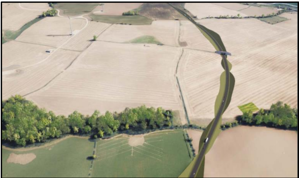
Figure 47 Extract from visualisation of Darlington Northern Link Road. Taken from Darlington Northern Link Road Brochure (Tees Valley Combined Authority and Tess Valley Mayor). Available at: https://teesvalley-ca.gov.uk/wp-content/uploads/2020/12/DNLR-Brochure-Design-Web-version-1.pdf
