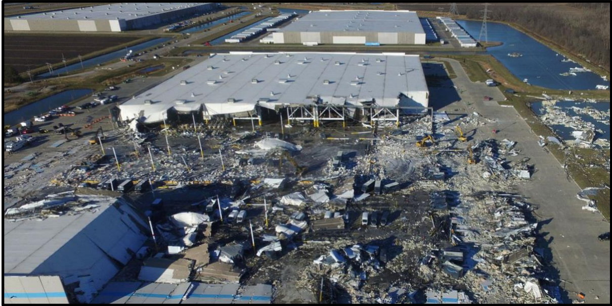
Figure 26 The site of a roof collapse at an Amazon.com distribution centre a day after a series of tornadoes dealt a blow to several US states, in Edwardsville, Illinois, US December 11, 2021. REUTERS/Drone Base. Available at: https://www.reuters.com/markets/commodities/amazon-driver-died-bathroom-sheltering-tornado-with-colleagues-2021-12-12/
