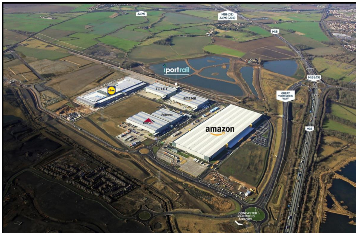
Figure 9 1.1 million sq. ft & 215,000 sq. ft Amazon warehouses in 'iPort', an Inland Port intermodal rail terminal in Doncaster, South Yorkshire. Published 2020, via iPort: Overview. Available at: https://iportuk.com/overview/
