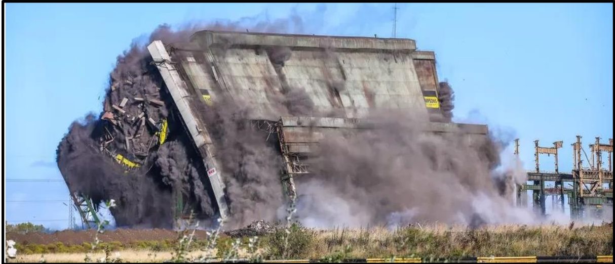
Figure 25 The levelling of the BOS plant at Redcar steel plant in October, 2022. Up to 1.6 tonnes of explosives was used to level the 65m (213ft) structure, which contained an estimated 105,000 tonnes of steel. BBC News . Available at: https://www.bbc.co.uk/news/uk-england-tees-63077791
