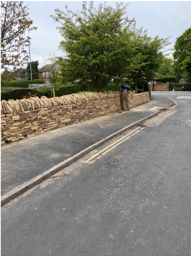
Fig. 5. The completed job.
