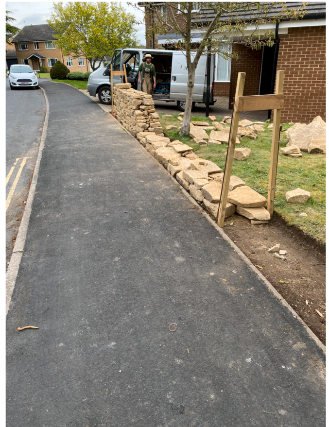
Fig. 4. Building the Wall in 6 m sections.
