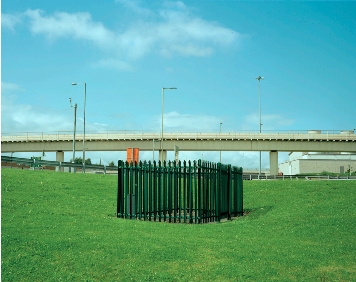
54.97723, -1.47956 Enclosure, A19 Facing North, 2017
