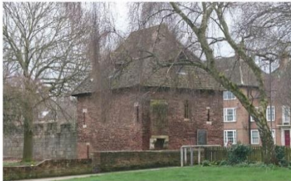
The Red Tower - an important but later circle
