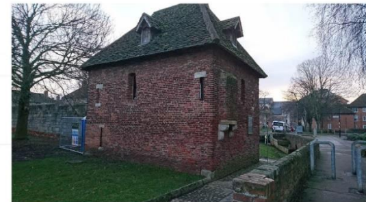
Distribution point for aterials during the Boxing Day floods
