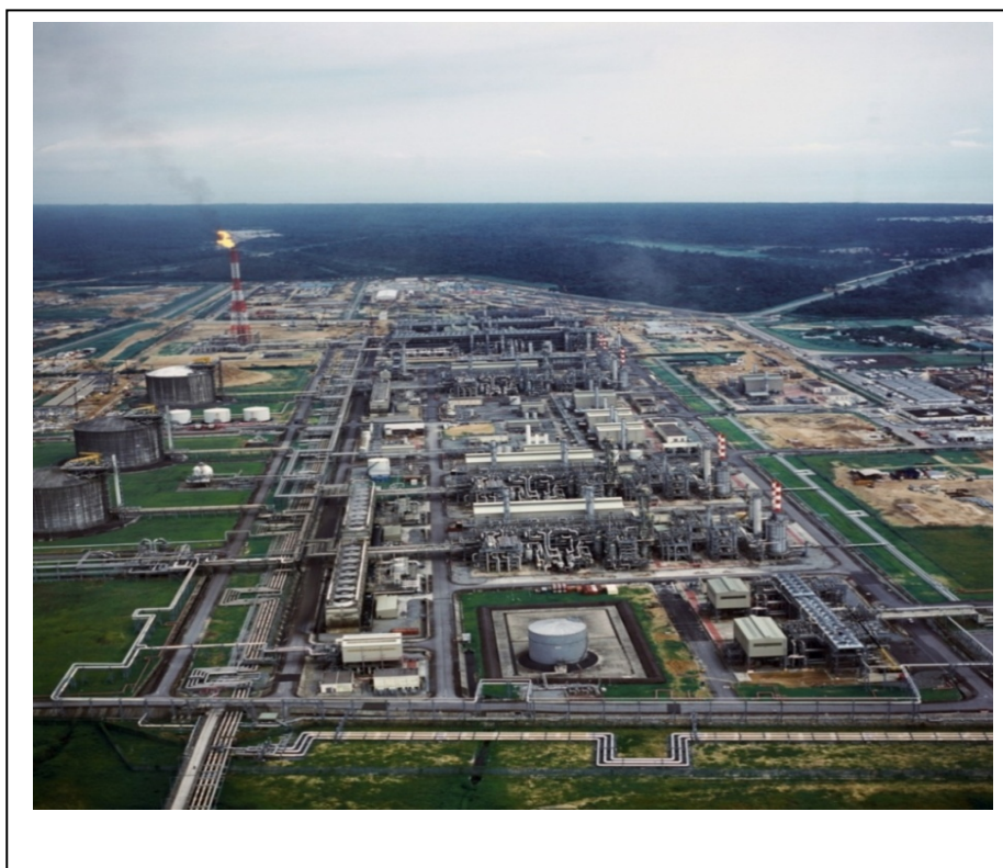
PLATE 1: The Nigeria Liquefied Natural Gas Project Complex
