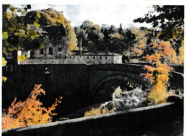
Aysgarth Falls Bridge
