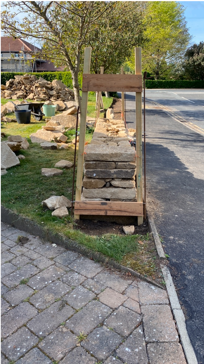
Fig. 3. Erection of batter boards.
