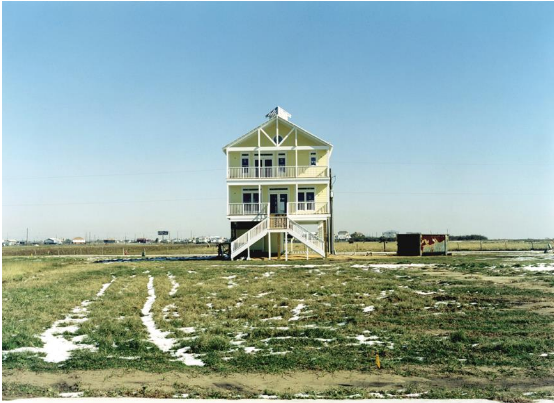
Land Development Site #02, Galveston, Texas, USA. Photographic Chromogenic Print of a luxury house on a housing construction site on the island of Galveston, Texas. (Edition of 50). 16x20 inches
